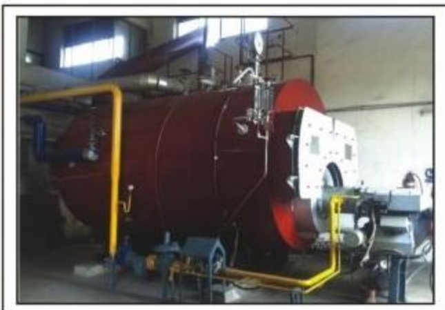
05 TPH @ 10 Bar (G) Smoke Tube Fired Steam Boiler
