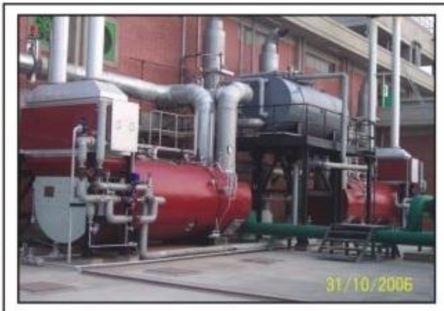
1.6 TPH @ 10 Bar (G) Waste Heat Recovery Boiler
