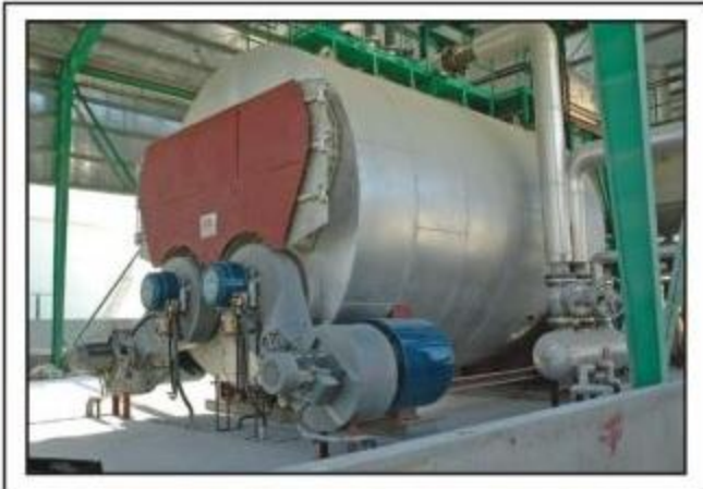
31 TPH @ 12 Bar (G) Smoke Tube Fired Steam Boiler
