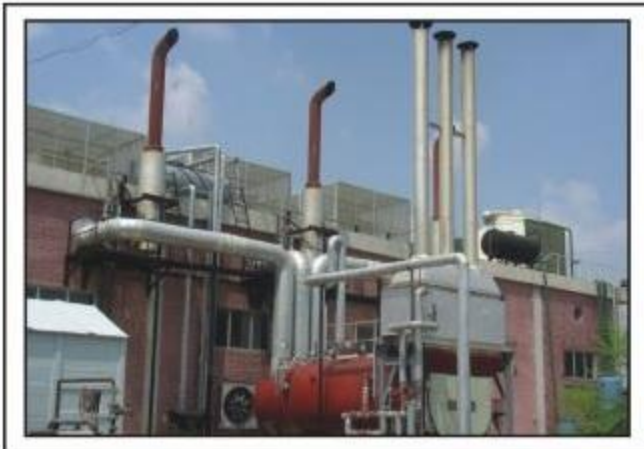
2.85 TPH @ 10 Bar (G) Waste Heat Recovery Boiler
