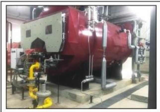
04 TPH @ 10 Bar (G) Smoke Tube Fired Steam Boiler
