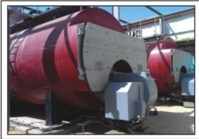
10 TPH @ 10 Bar (G) Smoke Tube Fired Steam Boiler
