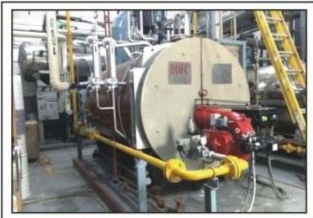
01 TPH @ 07 Bar (G) Smoke Tube Fired Steam Boiler
