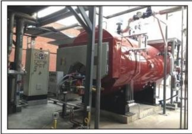
3 TPH @ 10 Bar (G) Smoke Tube Fired Steam Boiler
