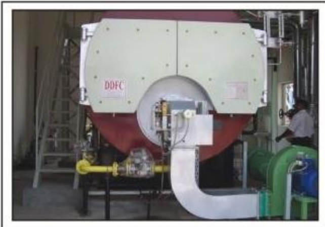
08 TPH @ 10 Bar (G) Smoke Tube Fired Steam Boiler
