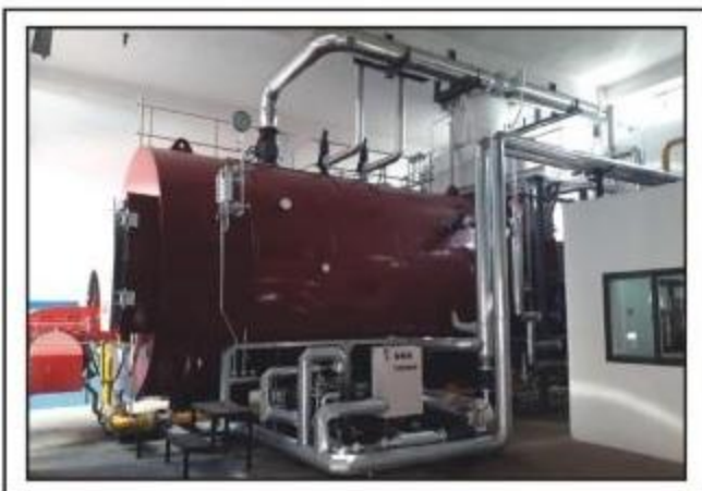
20 TPH @ 10 Bar (G) Smoke Tube Fired Steam Boiler
