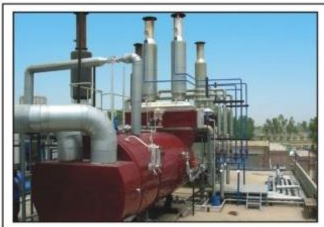
1.9 TPH @ 10 Bar (G) Waste Heat Recovery Boiler
