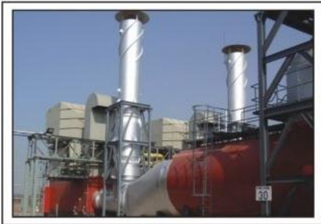
18 TPH @ 20 Bar (G) Waste Heat Recovery Boiler
