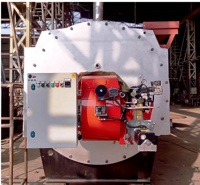
FIRED HOT WATER GENERATOR CAPCITY 288 US GPM @ 5.50 Bar (G)
