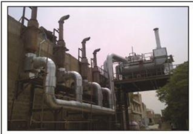
7.65 TPH @ 10 Bar (G) Waste Heat Recovery Boiler
