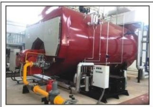
15 TPH @ 10 Bar (G) Smoke Tube Fired Steam Boiler
